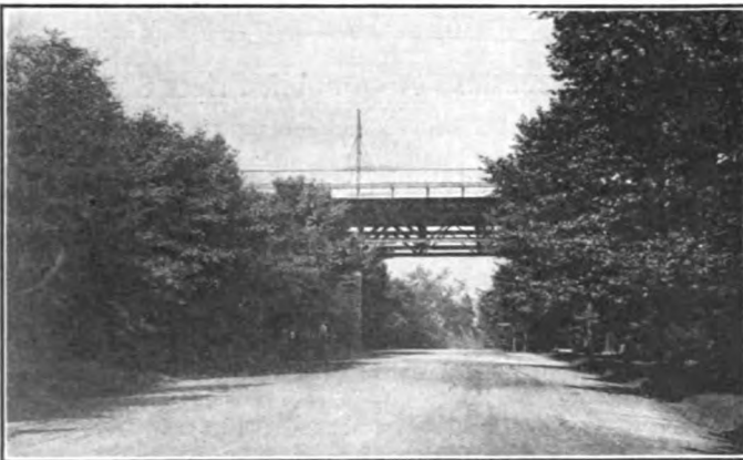
Under Strawberry Bridge on West River Drive
